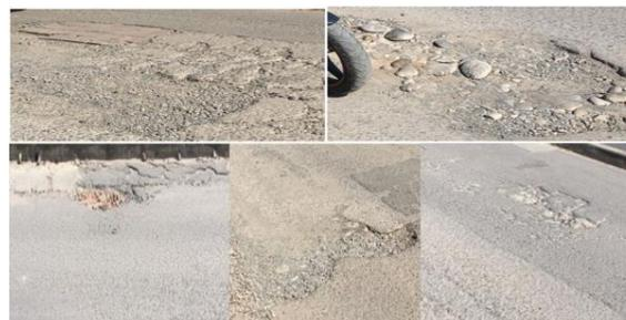
**Gambar 1. Kerusakan Jalan Tipe granular release, patches and potholes**
