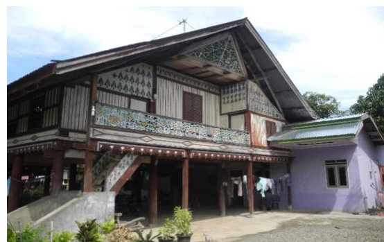
Figure 2. Side View of Rumoh Aceh with a Concrete Structure Added to the Lower Section
