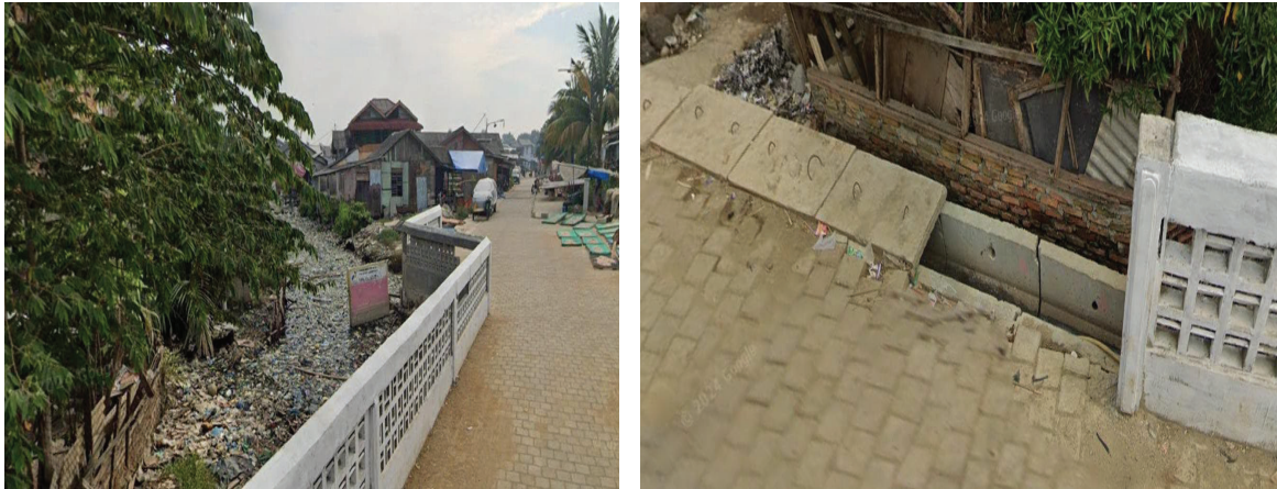
Figure 4. Drainage condition in a High-Density Residential Settlement
