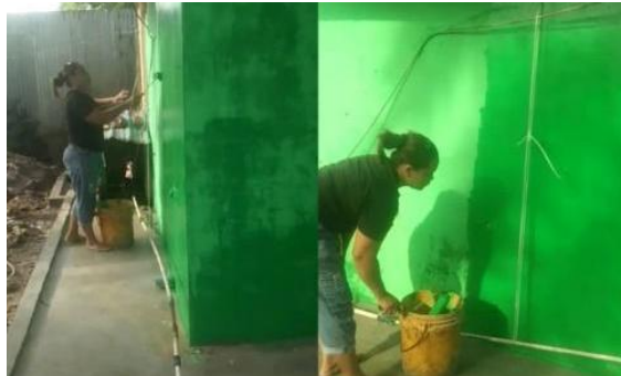
Fig 9. Process painting process of public bathroom.
