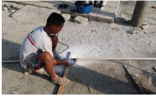
Fig 7. Cutting PVC pipe as many as 20 rods.
