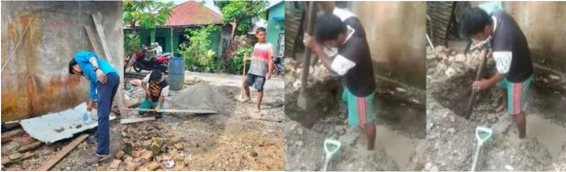
Fig 8. The process of making a septic tank.
