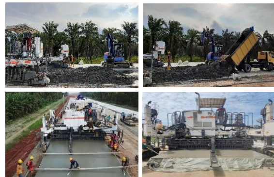
Gambar 14. Pengecoran rigid pavement
