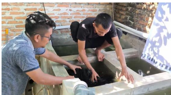
Gambar 5. Proses pengisian filter biologis dan mekanis
